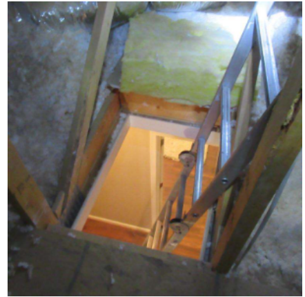
Image 3.4.3 Entry to Attic
