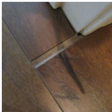
Image 6.1.1 Hardwood Flooring Gap - Master Bdrm Entry
